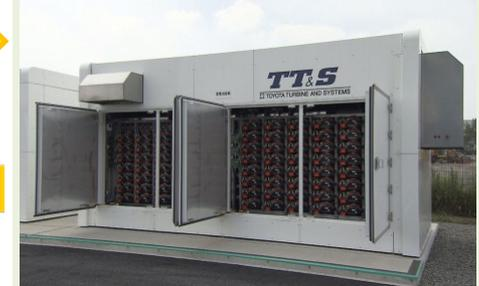
A rechargeable battery system reusing used batteries of hybrid cars is installed. Even when wind power is not enough, stable hydrogen production and supply are possible.
