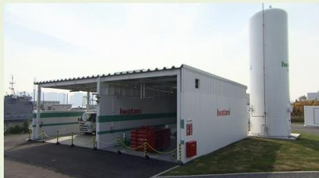
Hydrogen for 2 days is stored for stable supply of hydrogen. The tank's hydrogen is pressurized by the compressor and loaded into the fueling truck.
