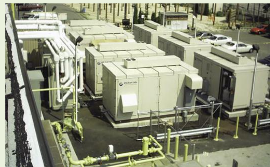
Seven UTC 200 kW PAFC installed at Verizon
