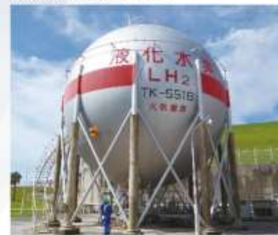
Type Spherical double-shell tank Storage Volume 540m 3
