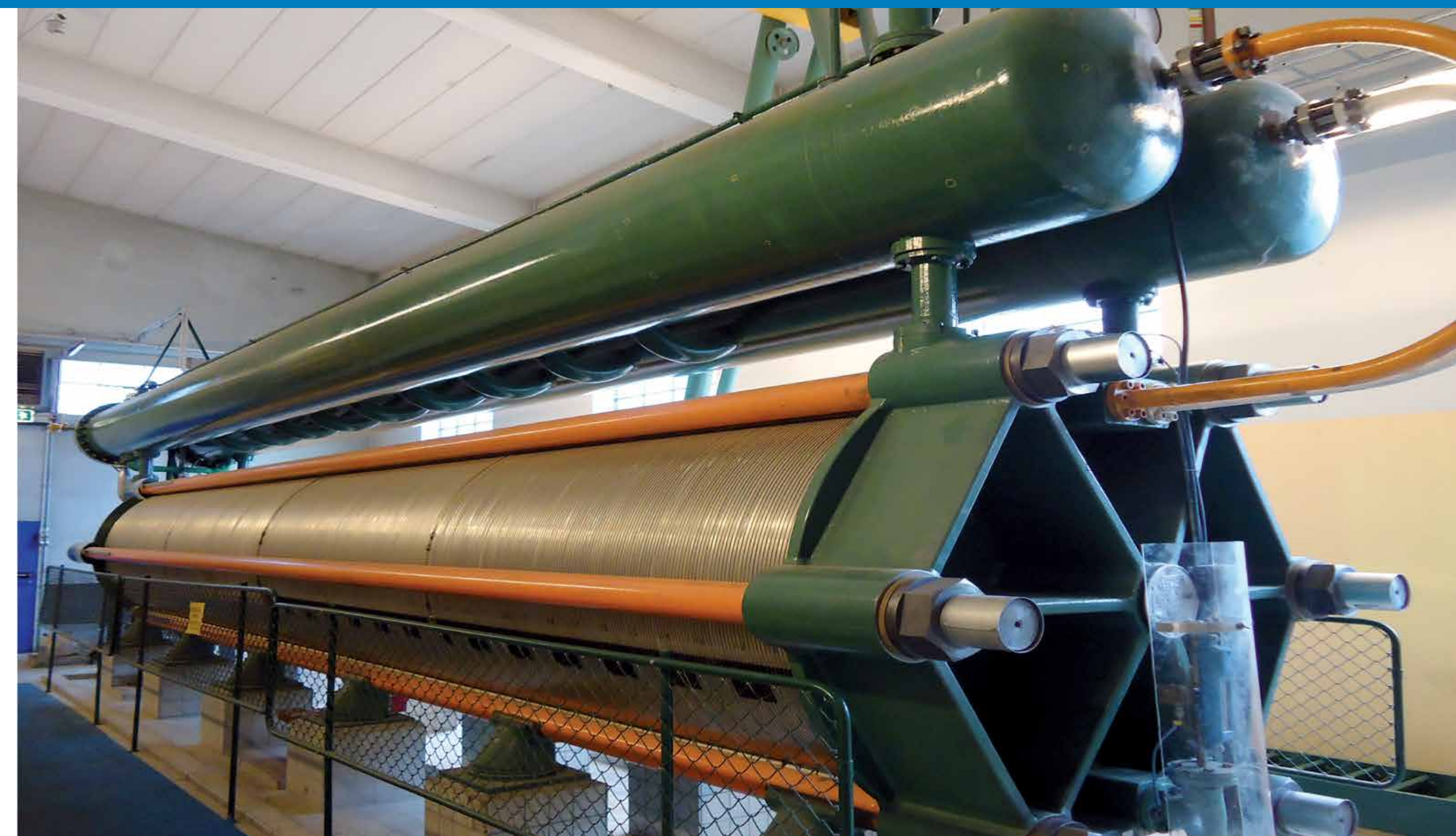
IHT Electrolyser – (760Nm 3 /h H 2 )
