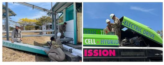
Interns from group 4 of the Hydrogen School being trained on maintenance of the H70 hydrogen dispenser (left) and conducting cooling system checks on one of the donated fuel-cell electric buses (right)
