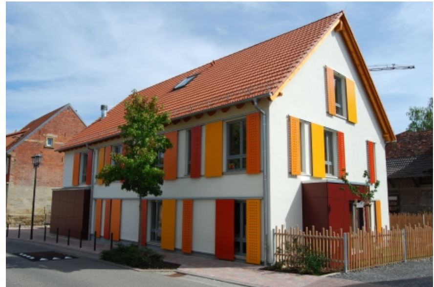
Day-care facility in Oberderdingen (Baden-Württemberg)
