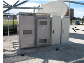
After installation of Fuel Cell
