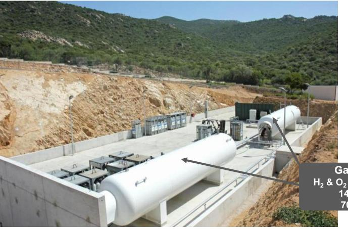
Gas Storage H<sub>2</sub> & O<sub>2</sub> tanks@ 35barg 1400 Nm<sup>3</sup> H<sub>2</sub> 700 Nm<sup>3</sup> O<sub>2</sub>
