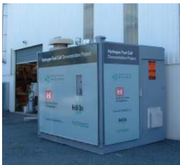
The housing at the US Antarctic Programme facility containing the methanol fuel tank, fuel cell system and monitoring equipment
