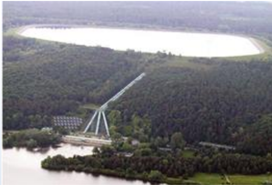
Geesthacht Pumped-storage Power Plant
