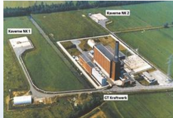
EON Huntorf CAES Plant
